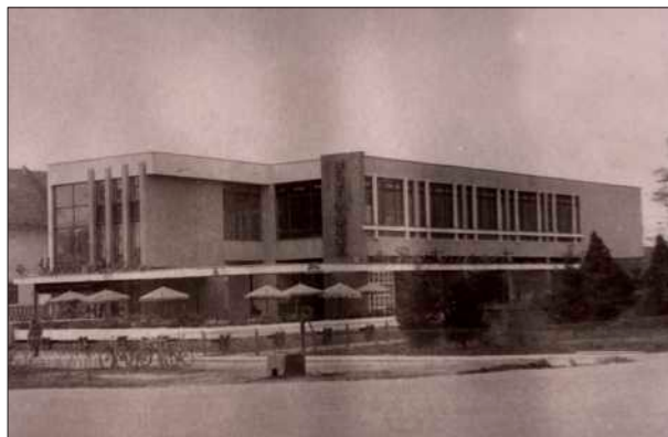
Complex de servire
